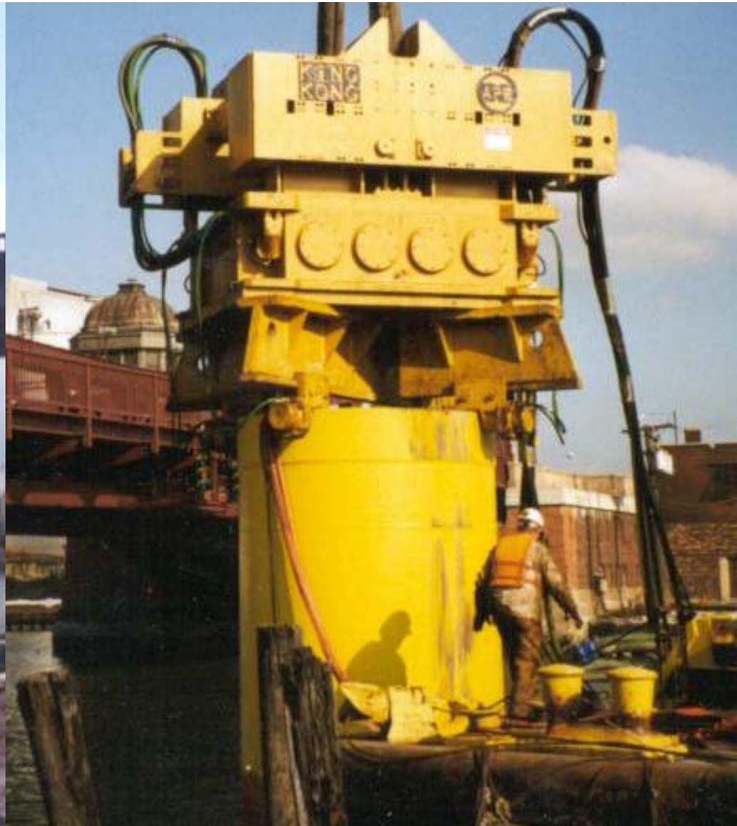
A vibro is a tool that, when attached to a pile, shakes it up and down in a vertical motion for the purpose of installing or removing it from the soil.
