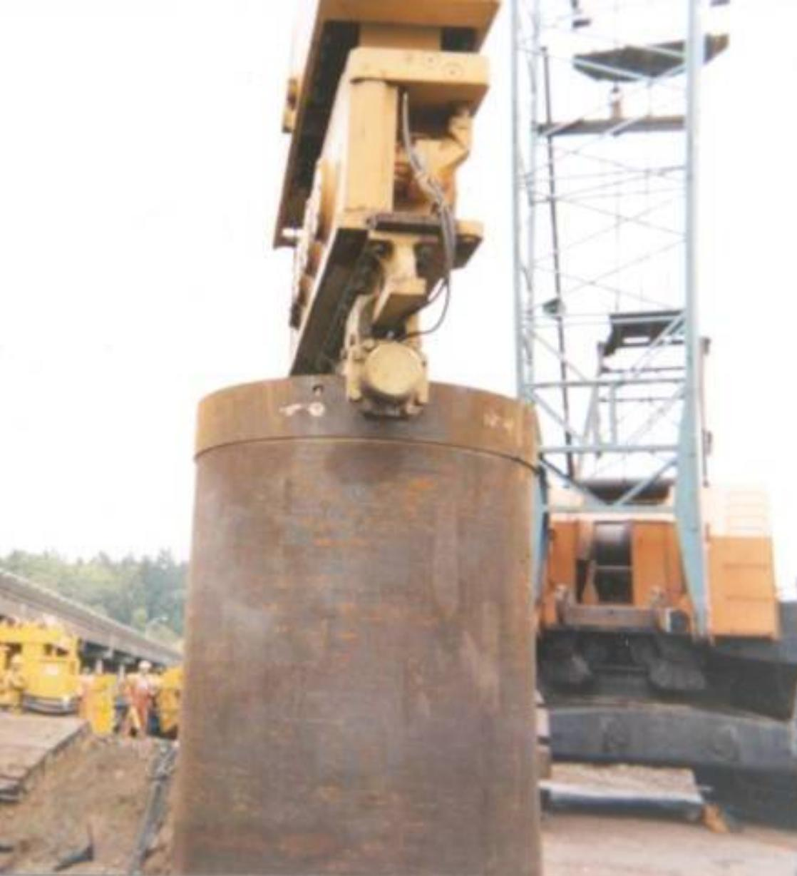
**Belly bands are added to the top and sometimes to the bottom of the casing to solve the following problems:**
